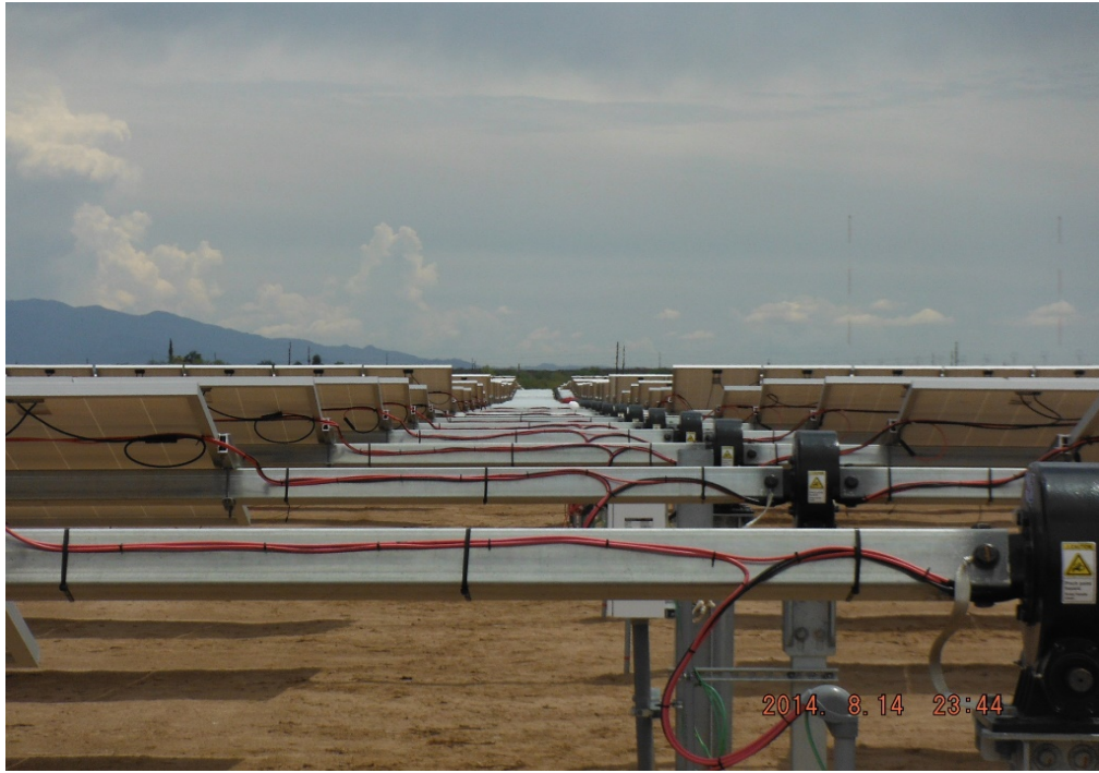
Figure 7 - Rows with completed module installation and string wiring
