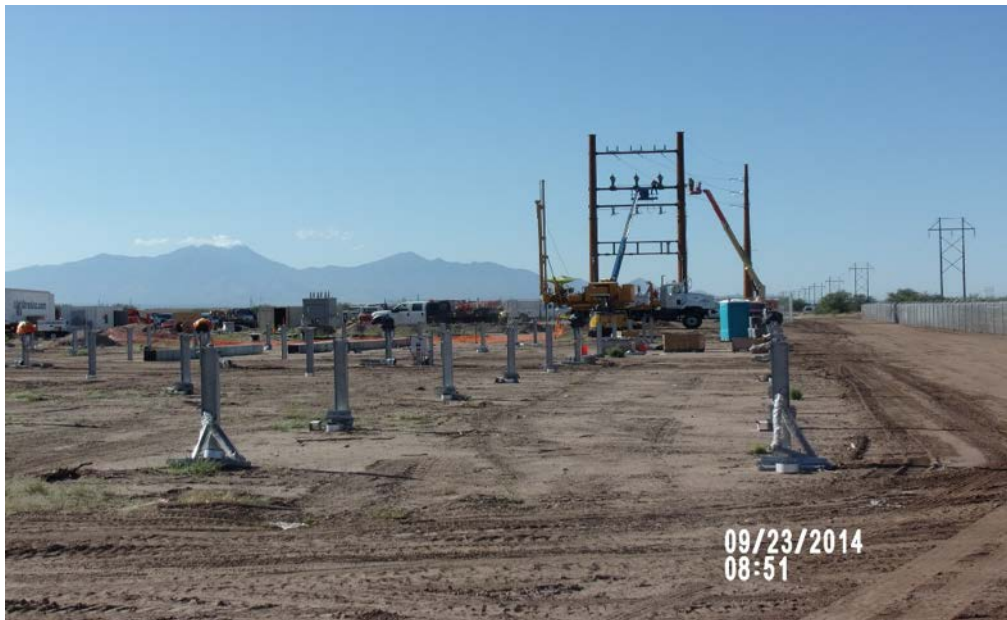
Figure 4 - Pile and Dead-End Structure Installation in Progress
