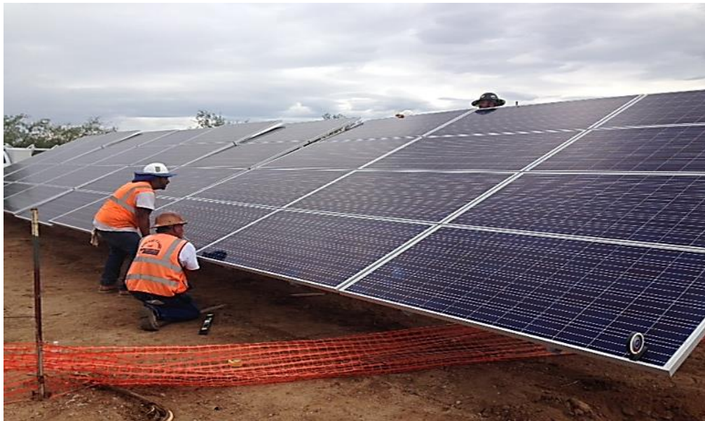
Figure 9 - Solar Module Installation at Mineral Discovery Center
