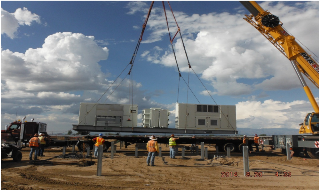
Figure 3 - Inverter Skid Installation in Progress
