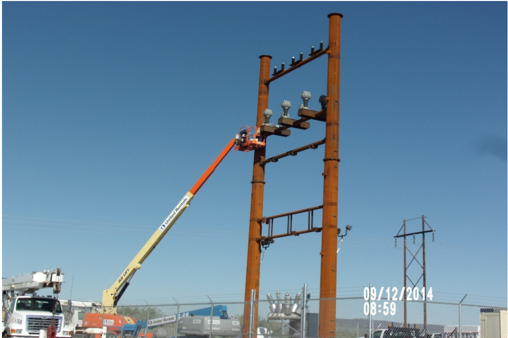
Figure 2 - Installation of Substation and Tucson Electric Power (TEP) Dead End Structure
