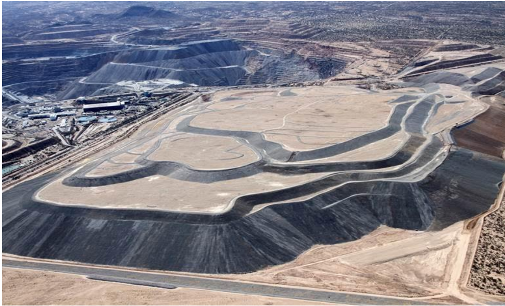
Figure 15 - Reclaimed Waste Rock Deposition Facility
