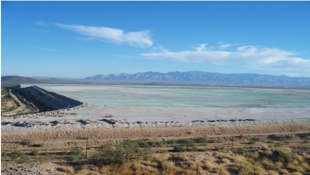
Figure 12 - Tailing Storage Facilities (TSF) before reclamation
