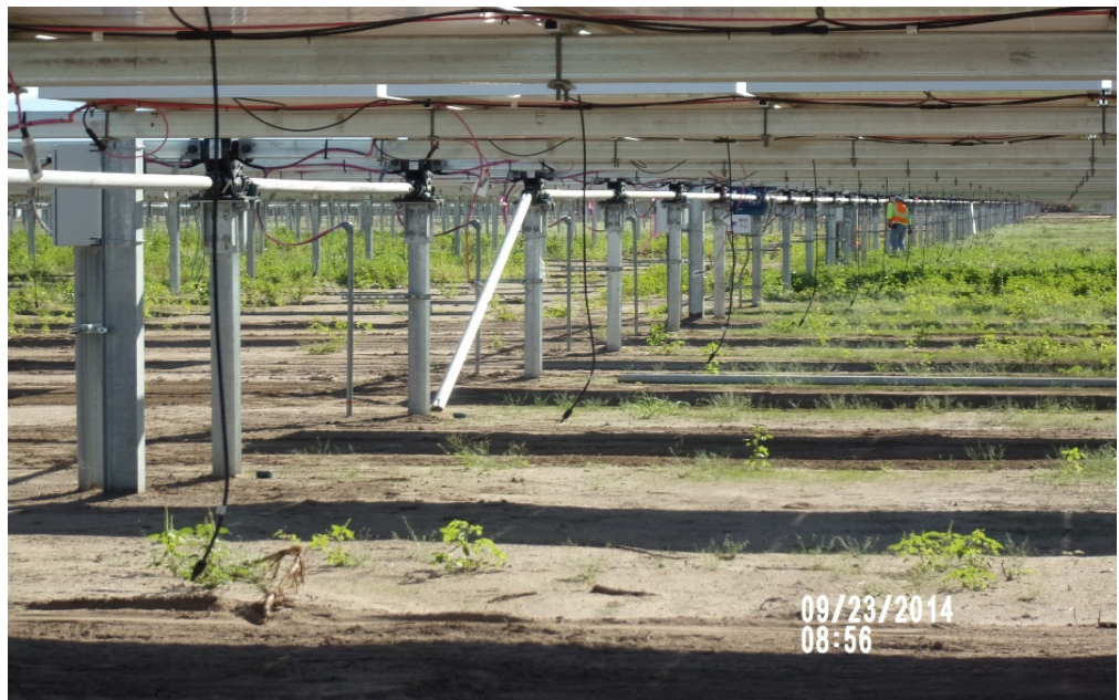
Figure 6 - Start of Stringing Wire Connections
