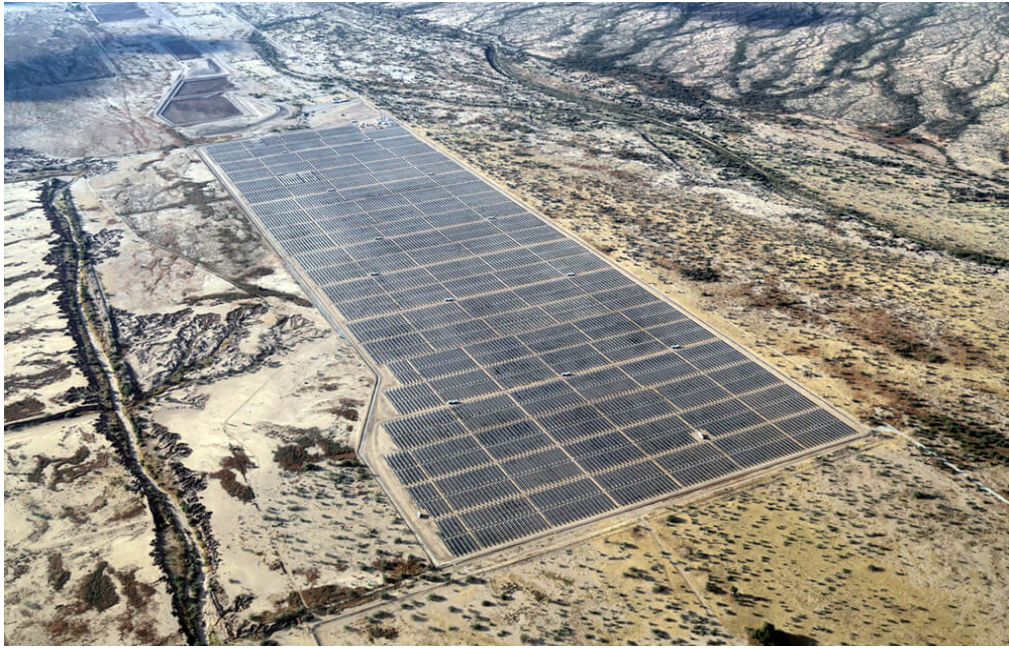
Figure 10 - Aerial View of the Avalon Solar Project
