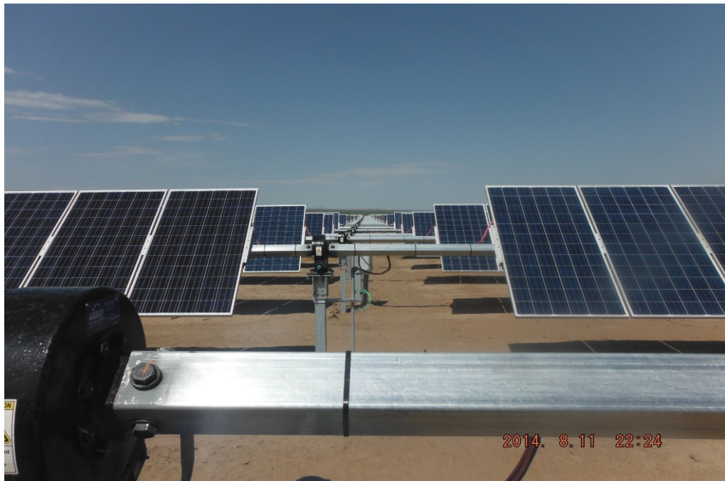
Figure 8 - Racking and Module Installed
