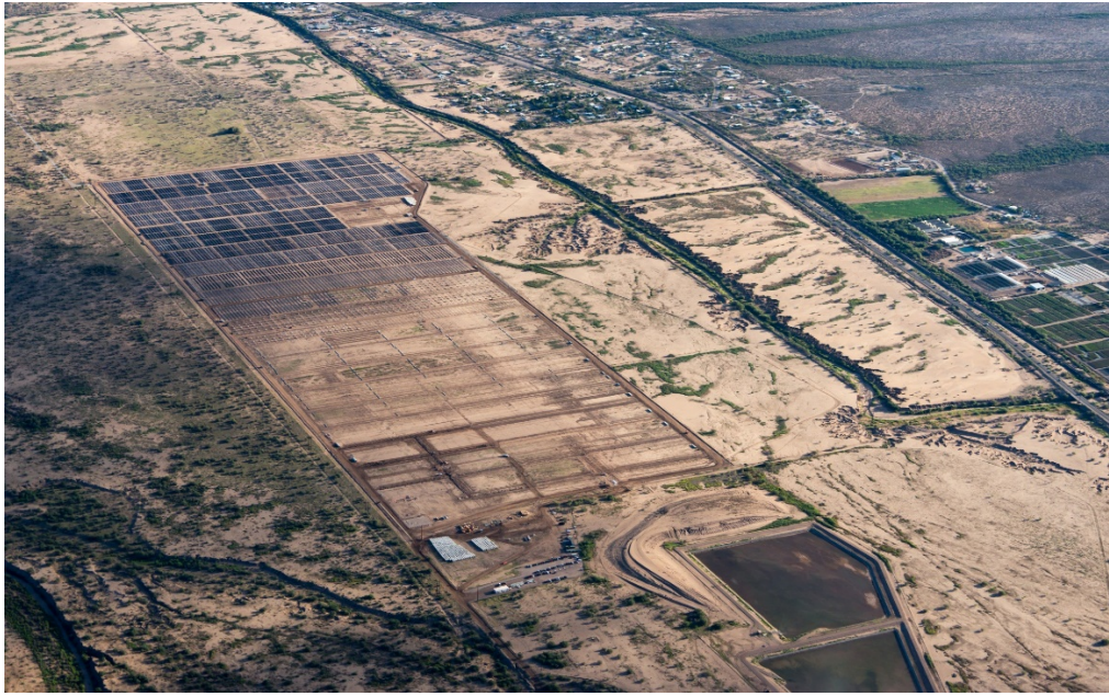
Figure 1 - Aerial View of Construction in Progress (9-14-2014)
