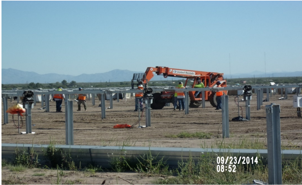
Figure 5 - Torque Tube Installation in Progress
